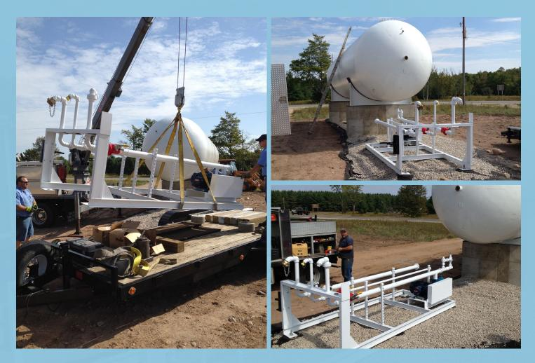
Lastly, we fitted the tank with RegO<sup>®</sup> internal valves, relief valves, and gauges. We then connected the piping on the tank to the piping skid. The entire on-site piping project took two installation technicians eight hours to complete.
