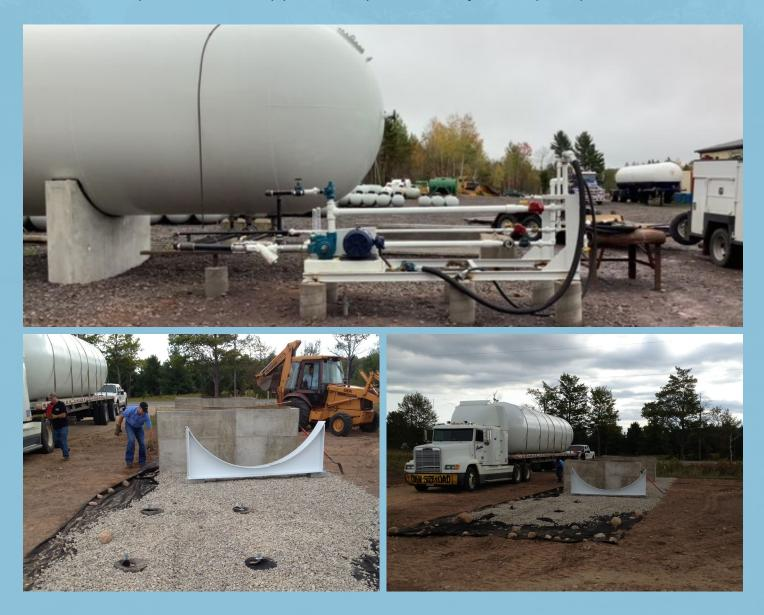
When we arrived at the job site, the concrete work was finished, allowing us to position the 30,000-gallon tank and the truck tightly against the supports.
